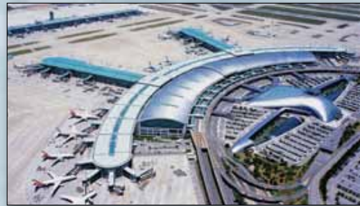
Incheon Airport Begins $4.6 Billion Expansion
