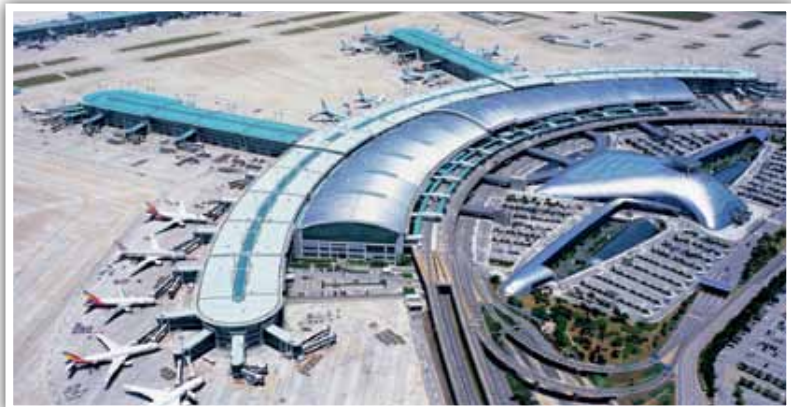
4) Incheon International Airport
